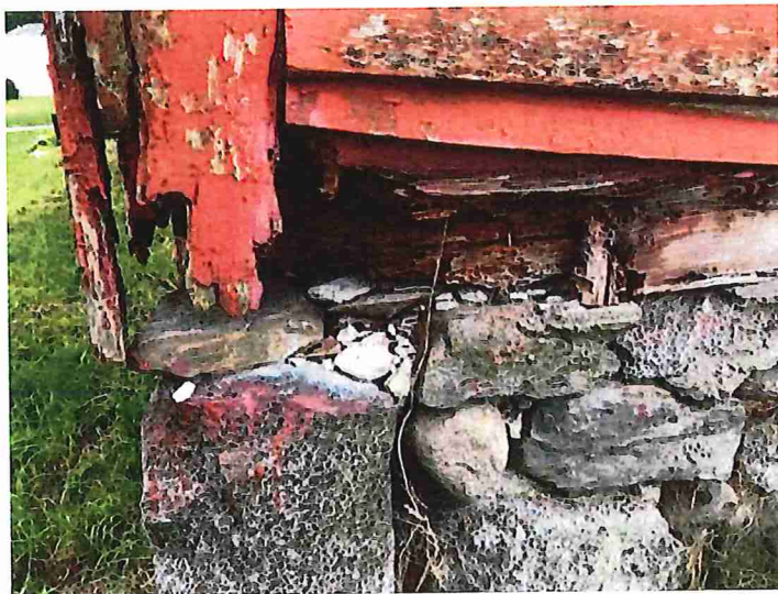
Figure 9 - Rotted sill, trim and clapboard at northeast corner of Storage Barn
