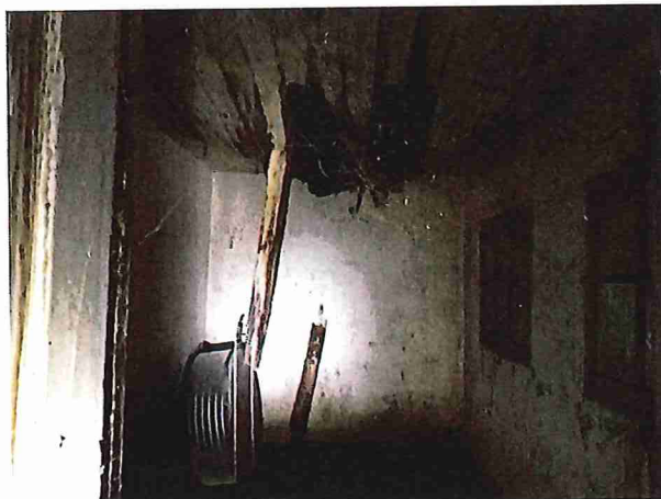
Figure 21 - Collapsed ceiling in small cooler (below Sawmill raised framing)
