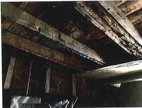
Figure 20 - Eastern sistered framing at Cellar showing rot, fire, and insect damage
