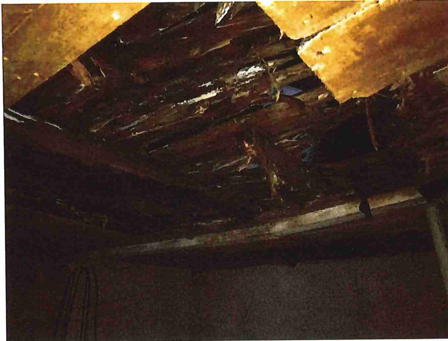
Figure 17 - Structural collapse over cold room. Note mid-span stop-blade scarf joint (splice) in beam (painted white), which is in failure
