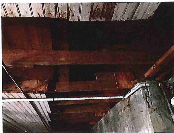
Figure 22 - Northern sistered framing, props and gussets, showing rot and insect damage
