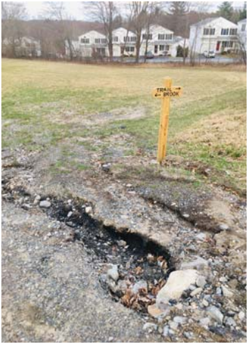
Runoff is eroding creating large ruts in the farm road, which is also part of the walking trail.
