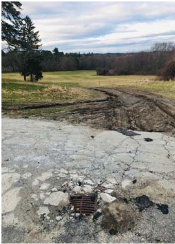
Erosion at top of the farm road, just beyond the drain at the base of the parking lot.
