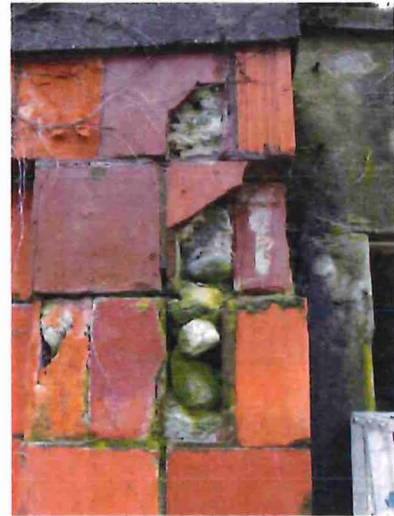
Figure 3 - rubble infill at northeast corner
