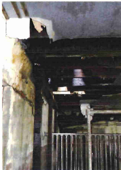
Figure 4 - collapsing joists at west wall
