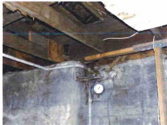
Figure 6 - north wall of cellar showing decayed joists & gussets & added post (photo right)
