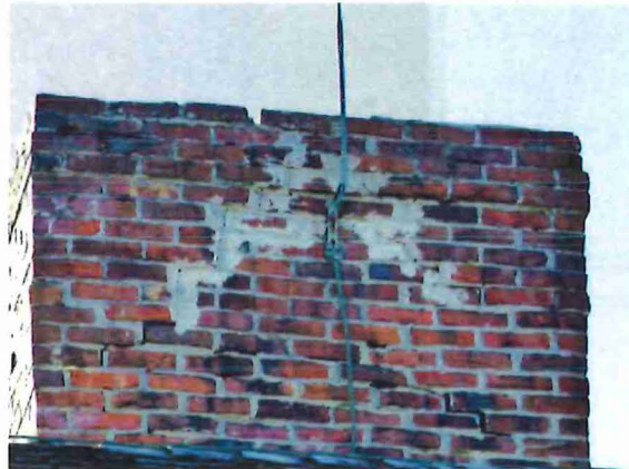
Figure 9 - north elevation of central chimney showing cracks & patches
