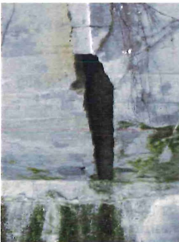
Figure 2 - corroding iron beam at ceiling
