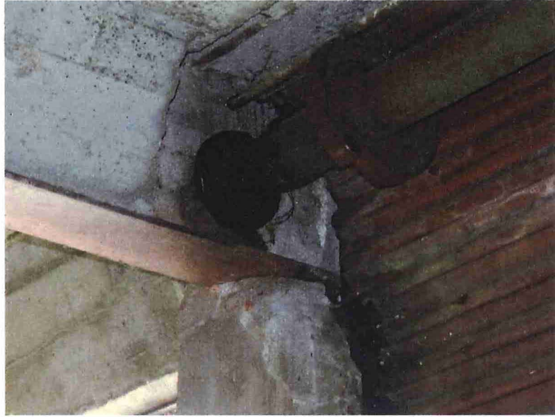
Figure 2 - detail of typical head of pier and steel beam at interior
