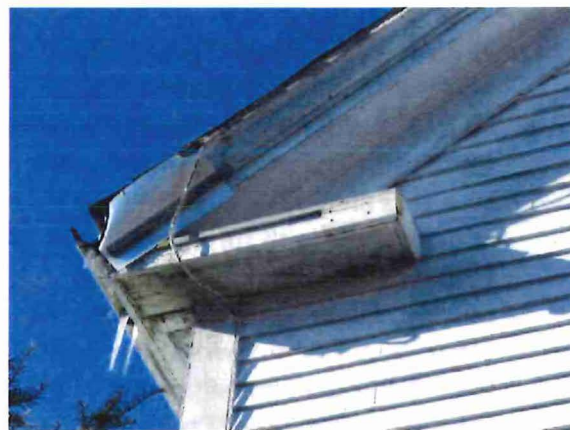
Figure 6 - main house - southeast corner with open gutter end & missing downspout
