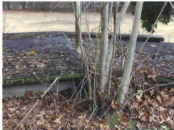
Figure 4 - trees growing through roof of corrugated cement asbestos
