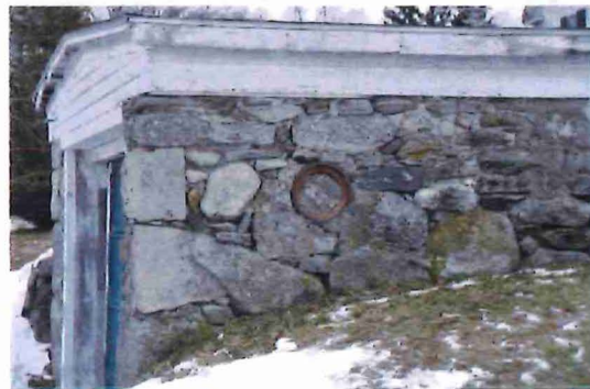
Figure 1 - north wall showing blocked terracotta pipe
