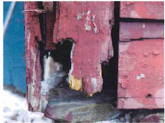
Figure 7 - deteriorated northeast corner post
