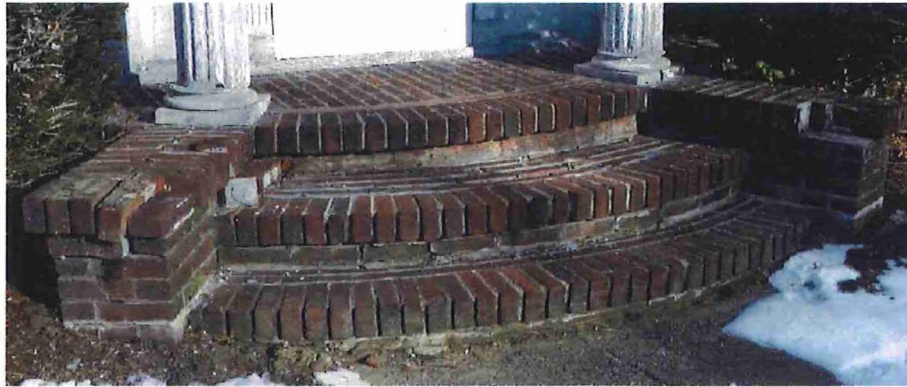
Figure 7 - damaged brickwork at front entry
