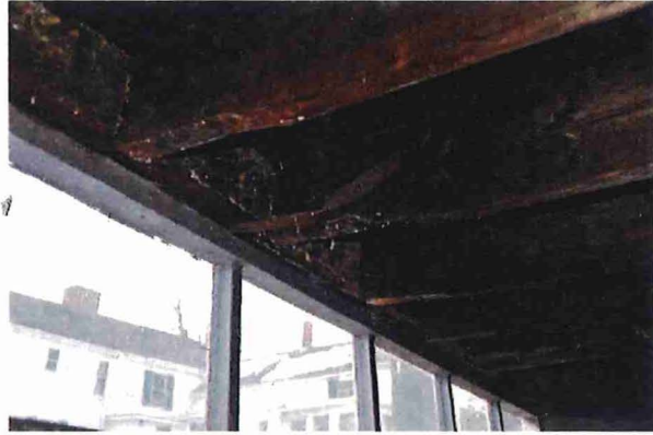
Figure 3 - roof framing showing possible frass caught in cobwebs
