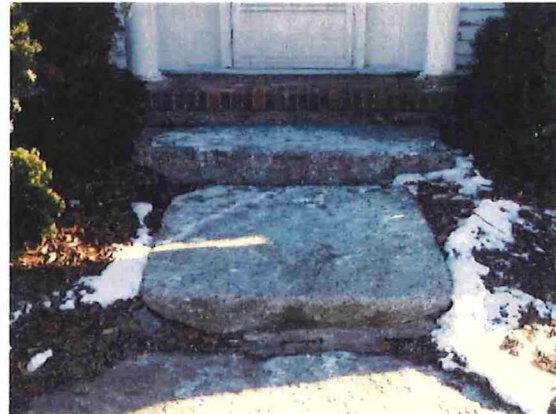
Figure 8 - west entry - granite steps re-set at ca. 1940 portico
