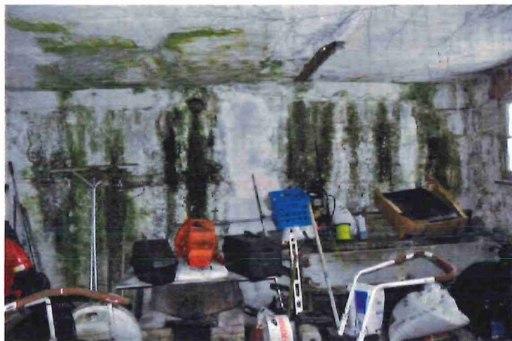
Figure 1 - algae, mold & vines at north wall
