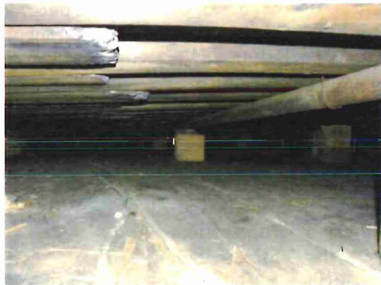
Figure 5 – roof structure & iron pipe on wooden blocks to stiffen roof
