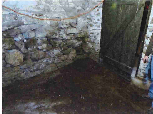
Figure 3 - south wall of main house foundation showing washed-out mortar joints & silt
