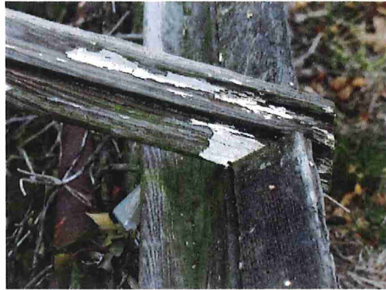
Figure 9 - mullion and internal gutter of greenhouse frame
