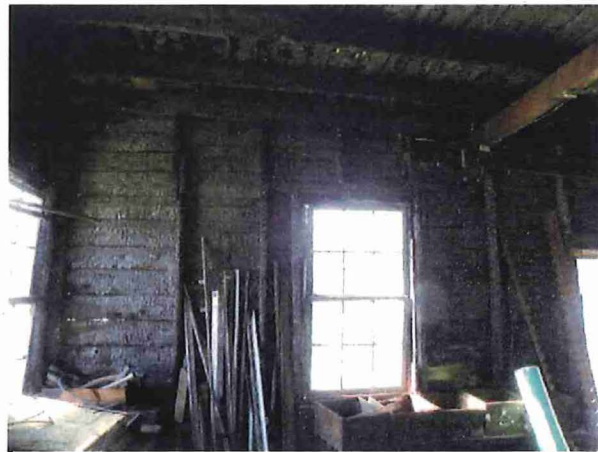
Figure 8 - southwest corner - charred framing
