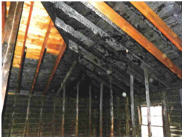
Figure 3 - southeast corner - fire damage from 1942
