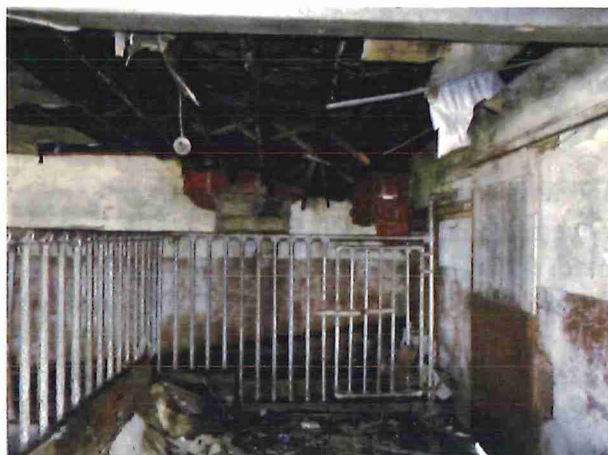
Figure 3 - northwest corner - collapsed joists
