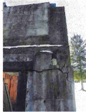
Figure 1 - typical cracked concrete at pier at Main Barn cellar
