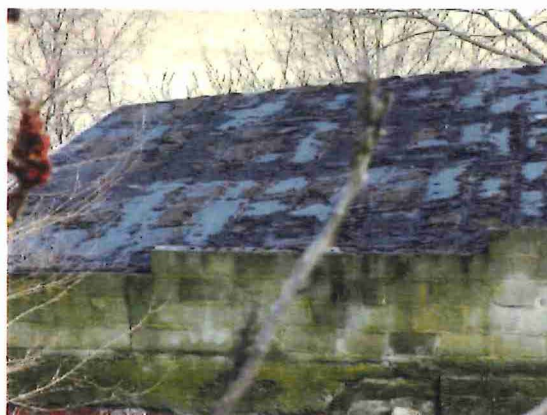
Figure 5 - rolled roofing at former base of Main Barn
