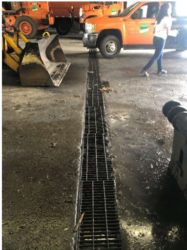
Floor Drain in Vehicle Maintenance Area
